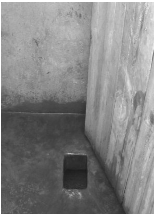
A typical pit latrine
